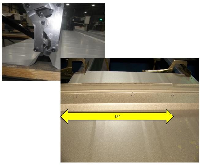
Below, is how the crimper should be aligned to start step 2 of the crimping process. During this step, you will push the release button on the back lever and pull it through the vertical arms until it bottoms out. This should only be done on the first 4" of the panel. Return the lever to the locked position. Do not remove crimpers from the seam at this time.
