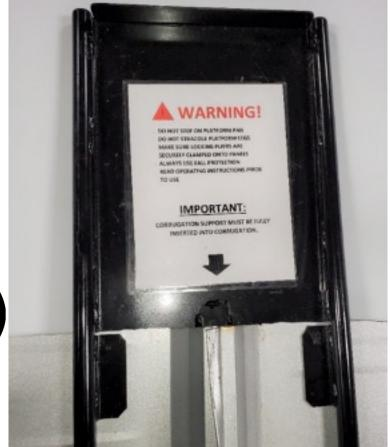
Ensure that the gate leg is engaged in the hole in the support tube as highlighted in the picture to the left. Lock clamps onto the panel as
