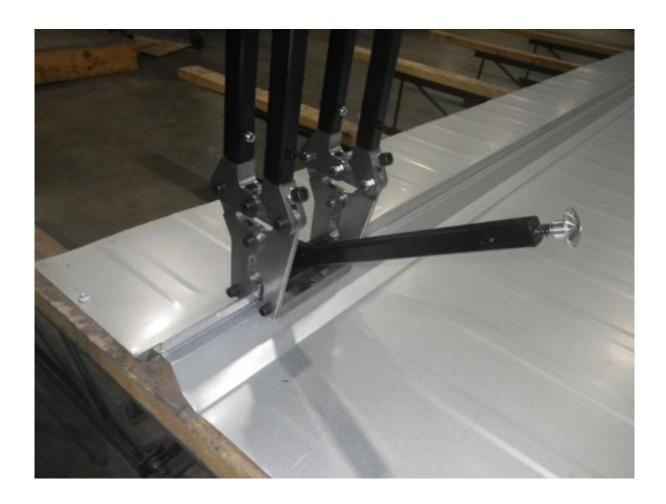
Once the crimpers have been removed place them back on the first 3 inches of the panel. Pull the vertical arms to the locked position to complete the 180° crimp and then remove the crimpers. This completes the crimping process for seamer engagement. The bottom photo shows how the completed hand crimp should look. Please note the measurements on the panel.
