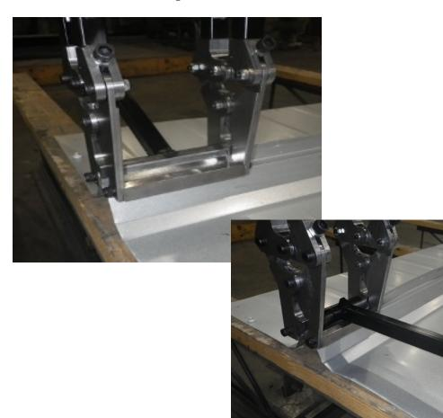
After releasing pressure on the lever, the crimper should be slid up the panel to the point where the panel has not been folded over from step 2. Press the release button on the back lever and pull the lever through the vertical arms to form a 90° bend on this portion of the seam. Return the lever to the locked position, open the vertical arms, and remove the crimpers being careful to not unfold the seam with the blade.
